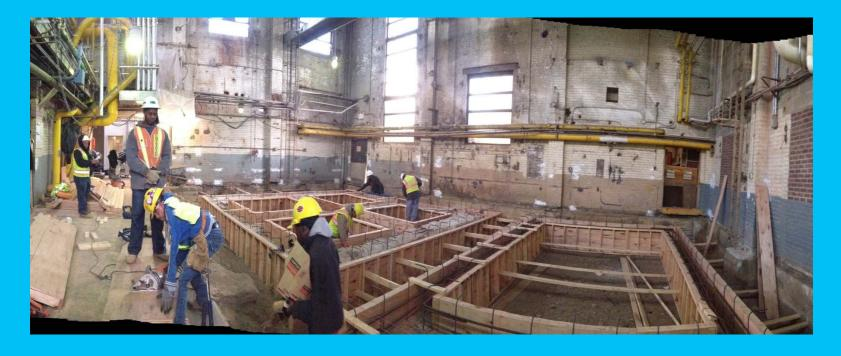
Structural repairs incorporating resiliency design of boiler room floor after damage from Hurricane Sandy .
