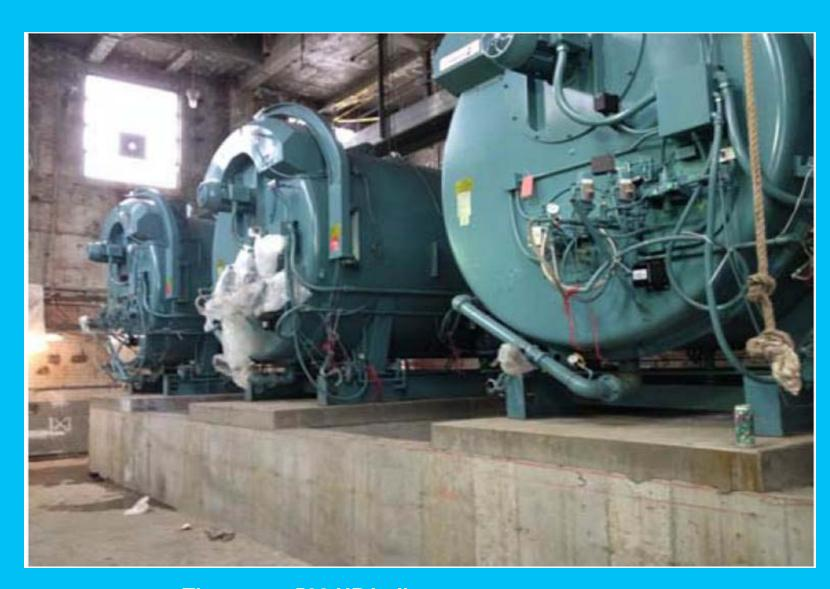
Three new 500 HP boilers on new supports.
