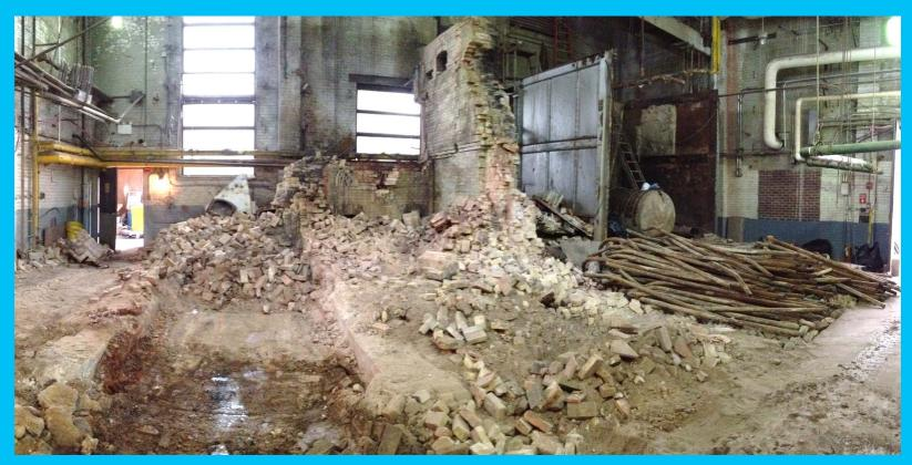
Post Sandy demolition of boilers installed in 1930's and 1950's
