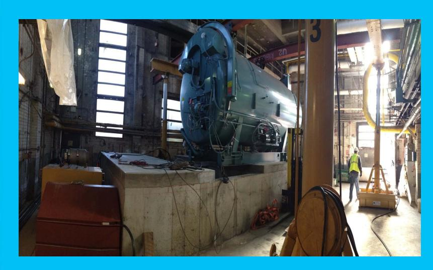
New boiler being rigged unto new support.
